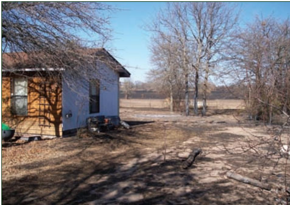
The lack of a break in fuels allowed the fire to burn directly to the side of the structure and melt the vinyl siding. The homeowners were forced to evacuate, but family members returned after the initial fire front passed to continue suppression efforts, saving the home.
