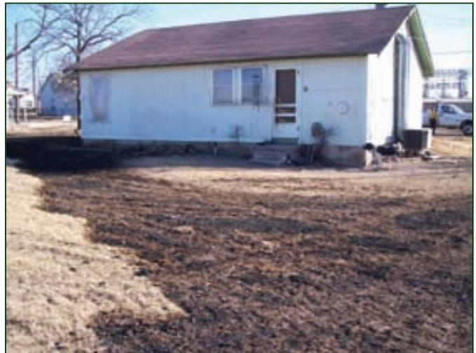
Dog runs on the front and back side of the home created a fuel break, keeping the fire from making contact on three sides of the home. Fire traveled to the side of the home where the dog's movement was restricted, allowing the fire to come in direct contact with the wood siding home. Radiant heat was significant enough to compromise single-pane windows and melted vinyl blinds.
