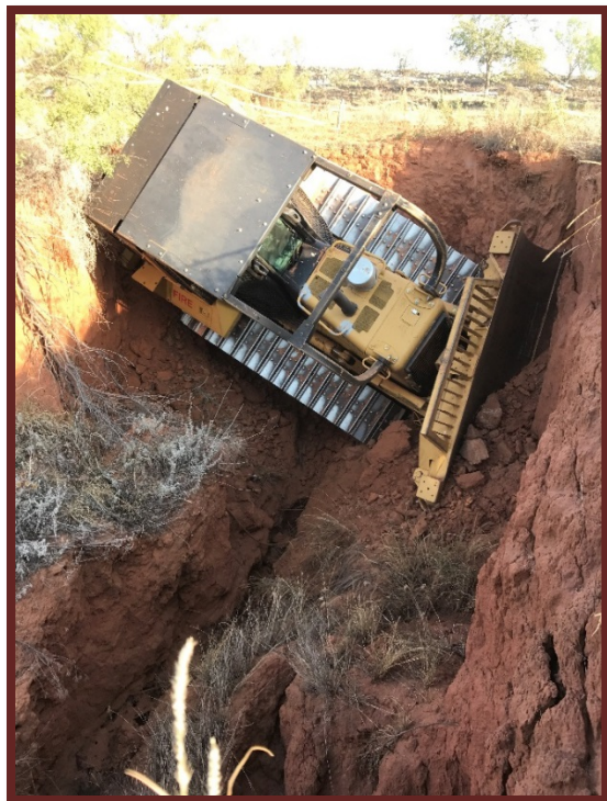
Looking up-drainage toward motor grader line
