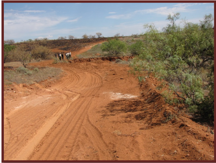
Looking down motor grader line, showing bend in the line around ravine (post dozer removal)
